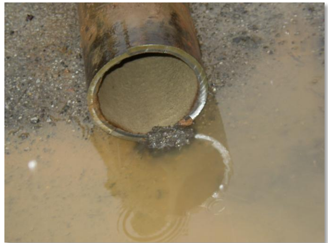
Pipe condition away from failure
