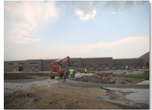
View of main building and paver installation
