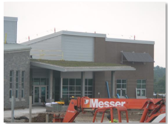
Vegetated "Green Roof"
