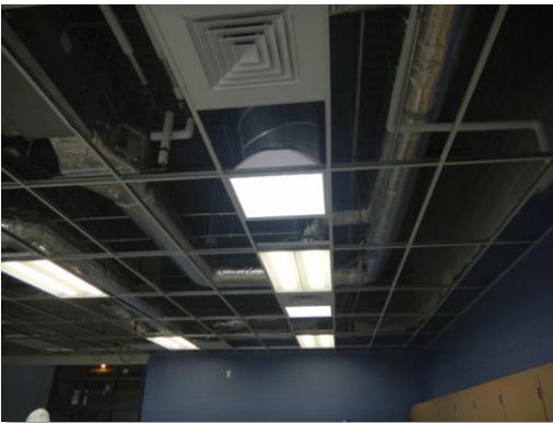
Classroom solar tube daylighting supplemented with T5 fluorescent lighting
