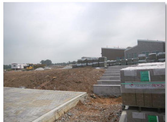
Exterior approach to the facility
