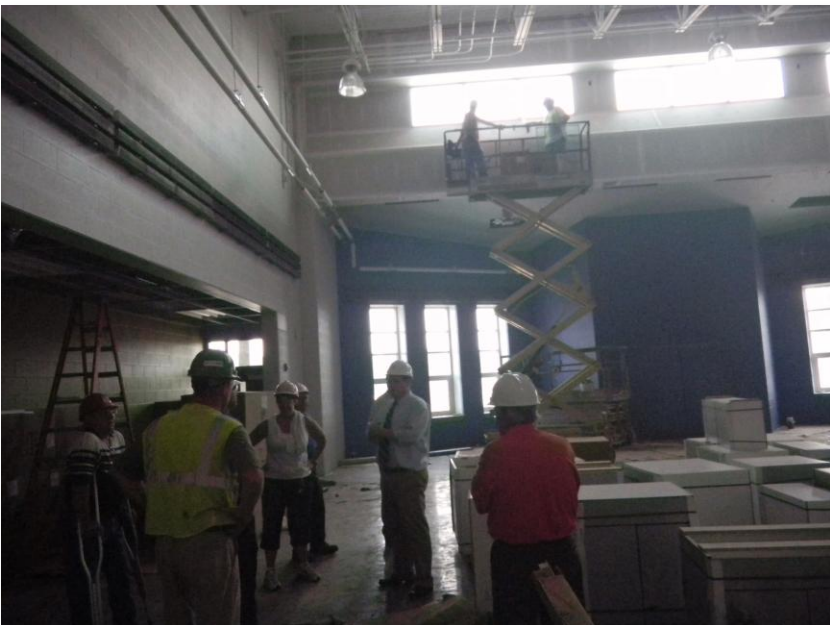
Interior work in progress
