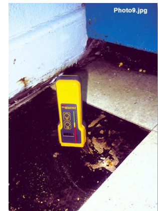
Moisture meter measuring moisture content of plywood subfloor
